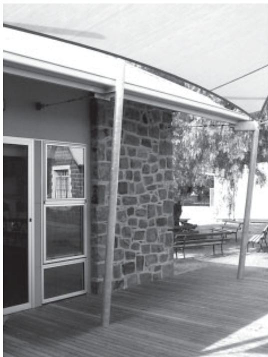
Figure 5. The blending of bluestone, double glazing, Ecoply and timber decking imbues a light restful ambiance that extends into the surrounding school grounds
