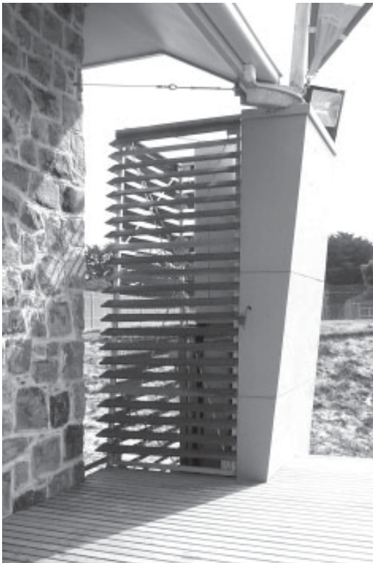
Figure 7. The heat pump is only required in the early morning and late afternoon
