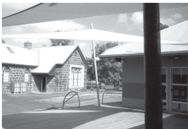
Figure 2. The existing bluestone building became an important aspect in the design of the redevelopment
