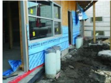
The intake ducts, taped off and yet to be finished off with cowls, adjacent to the school's external walls
